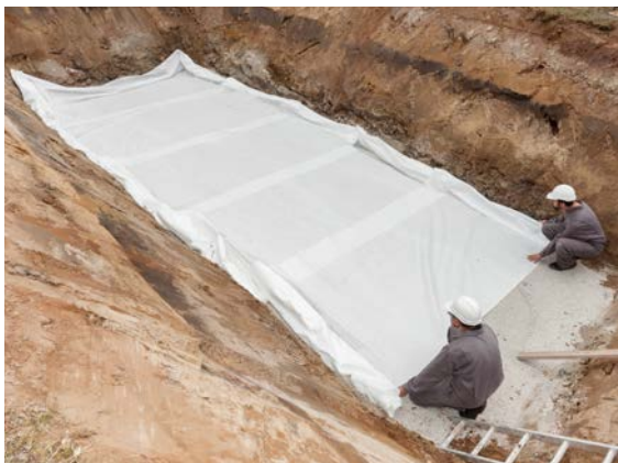
Prepared trench with RAUMAT geotextile filter
