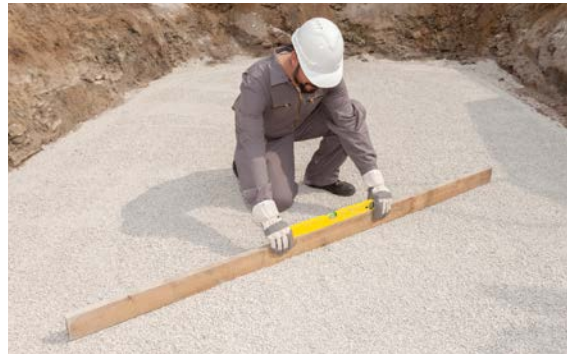
Prepared excavation pit.
